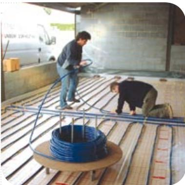
The plastic tube in the WTH Thermolink system has thick walls and is seamlessly extruded.
